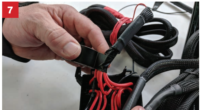
7 Use electrical tape to cover exposed red wires.
